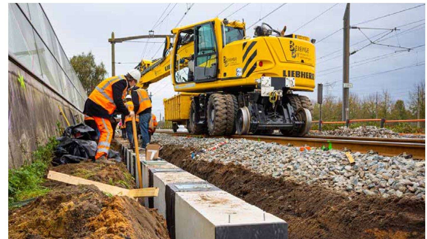
Figure 33 Installation of MetaBarrier
