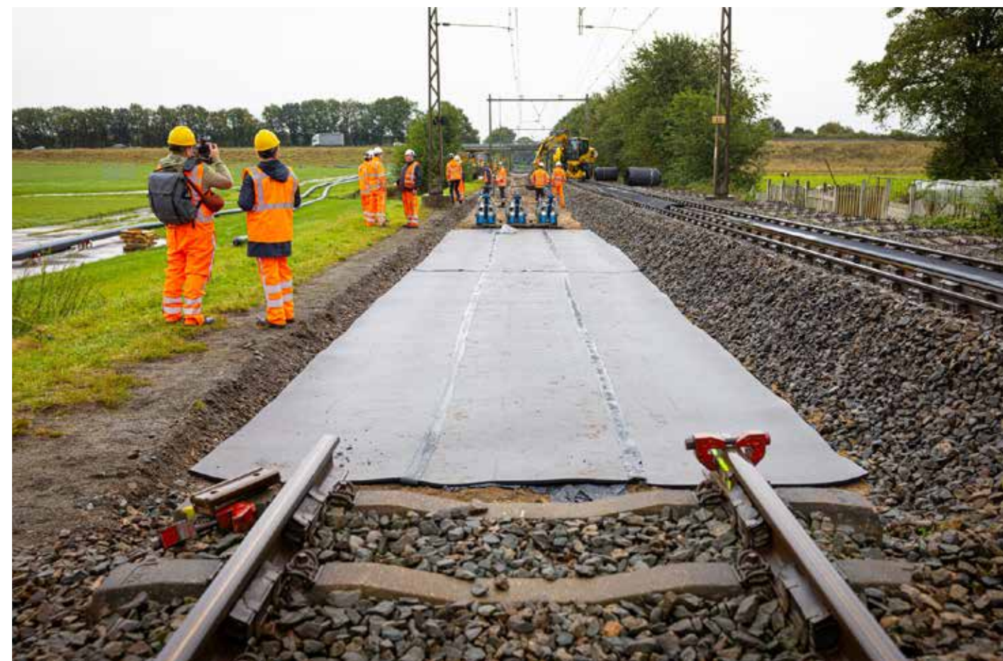
Figure 25 Installation of ballast mats at the test site
