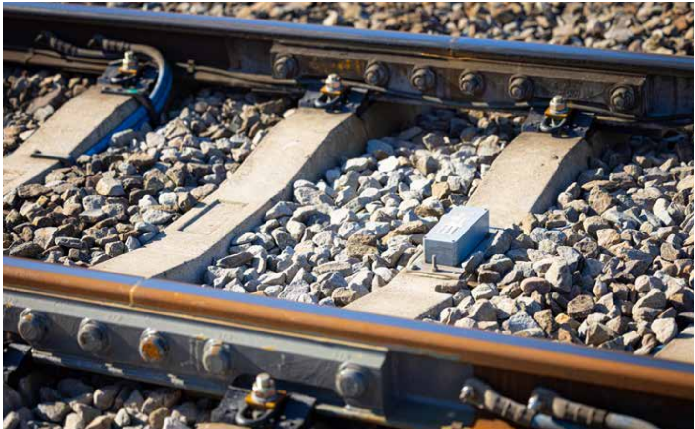
Figure 30 Photo of installed sensor – Adjustable IRJ
